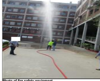
Photo of fire safety equipment Fire safety to confirm sustenance- Checking of fire hose.JPG
